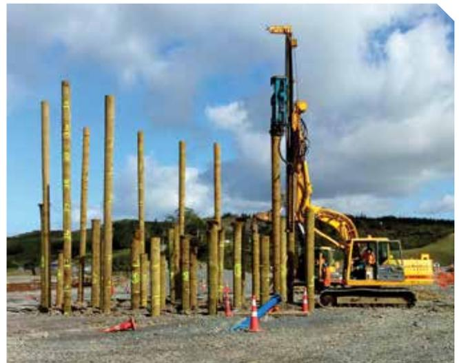
40 timber piles were driven up to 10m into the ground to support the fire water tank
