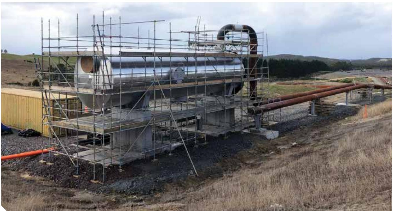
Geothermal fluid separator vessel installed and connection of steam line in progress
